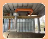
The carbon filter bed to remove odours from the air
